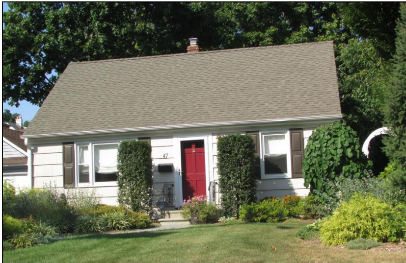
Figure 84 - This dwelling at 47 Columbus Avenue displays the Colonial Revival Cape Cod characteristics of symmetry with a steep roof, side gables and small overhang.
