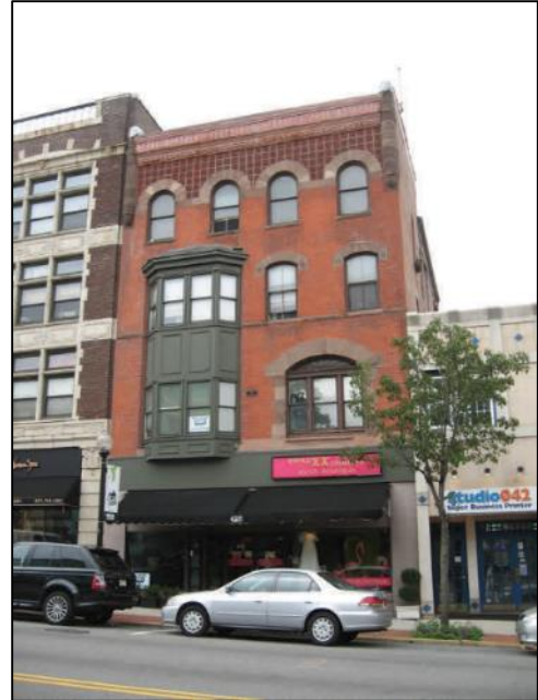
Figure 61 - Rounded arches and textured masonry are common features of the Romanesque Revival style (425 Bloomfield Avenue)
