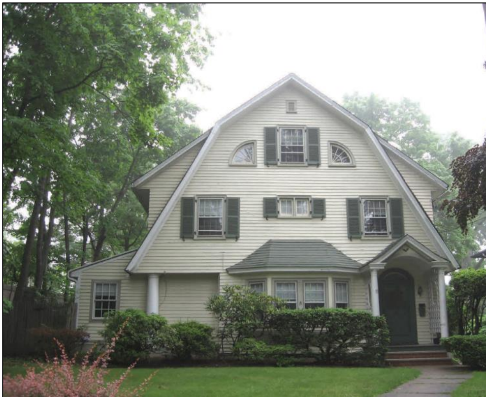
Figure 67 - This dwelling at 33 Fairfield Street was designed in the Dutch colonial style and features a prominent gambrel roof on the primary façade. The entry porch has Doric columns and at the roofline are shed dormers.
