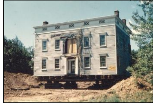
Figure 174 - The Israel Crane House was moved as a last resort to avoid demolition. A group of concerned citizens rescued it, and moved it to its new location on Orange Road.
