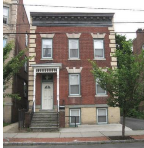
Figure 9 - Both residential and commercial properties are reviewed in the Pine Street Historic District (89 Pine Street)
