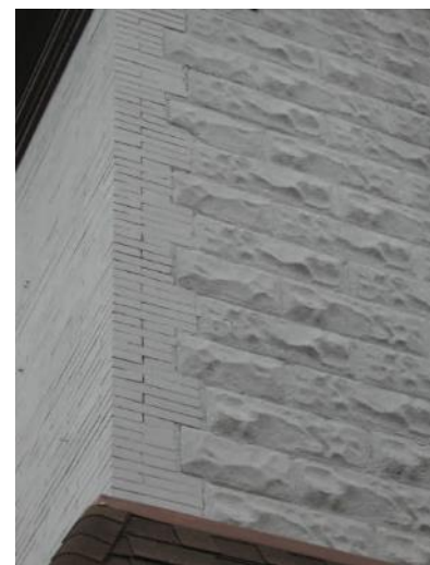
Figure 107 - Concrete block and brick masonry exterior at 613 Valley Road.
