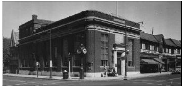
Figure 8 - Montclair's locally landmarked historic districts are composed primarily of commercial buildings such as in the Upper Montclair Historic District
