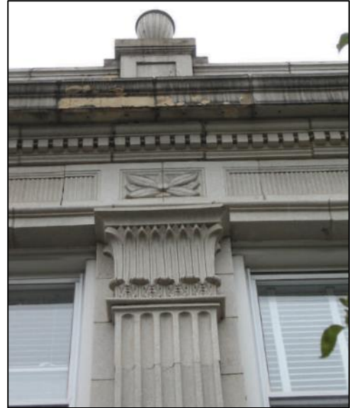
Figure 68 - The terra cotta details at 605 Bloomfield Avenue - fluted pilaster and capital, cornice dentils, and cap with urn - characterize the Neo-Classical style.
