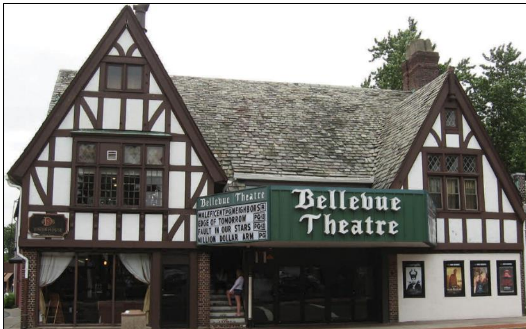
Figure 74 - The Bellevue Theatre on Bellevue Avenue represents the Tudor Revival style, with steep roof lines, a slate roof, and an exterior of stucco with half-timbering.
