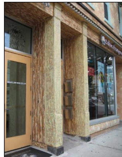
Figure 112 - Cast iron pilasters remain at this storefront at 440 Bloomfield Avenue
