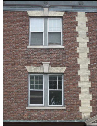
Figure 120 - Original six-over-one sash windows with brick jack arches at 598 Valley Road.
