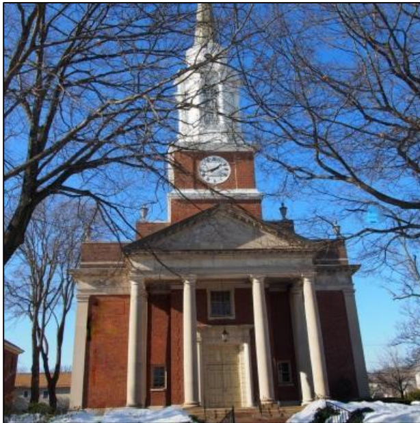
Figure 47 - Central Presbyterian Church at 46 Park Street was designed by the architectural firm of Carrère and Hastings, of New York, in 1921.
