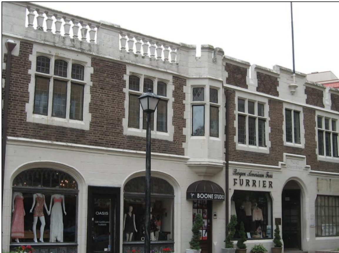
Figure 76 - The Hall Building at 40-46 Church Street was built in 1925 and designed by the architectural firm of Holmes & Von Schmidt. It is a rare example of a commercial building designed in the Collegiate Gothic style and has diamond-light windows and large, arched display window openings with metal decorative trim. The crenellated central parapet are high-style, character-defining architectural features of the style.
