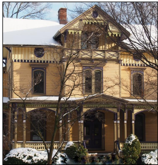
Figure 55 - A Carpenter Gothic influenced dwelling at 51 Park Street
