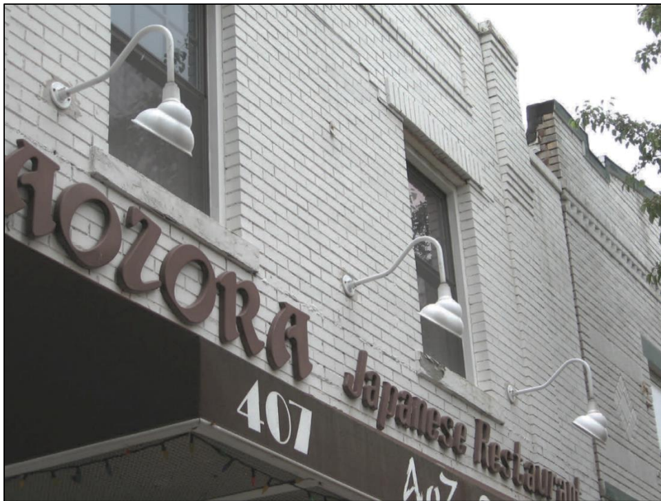
Figure 102 - Swan- or goose-neck fixtures in metal are appropriate new light fixtures for commercial buildings, as at 407 Bloomfield Avenue).
