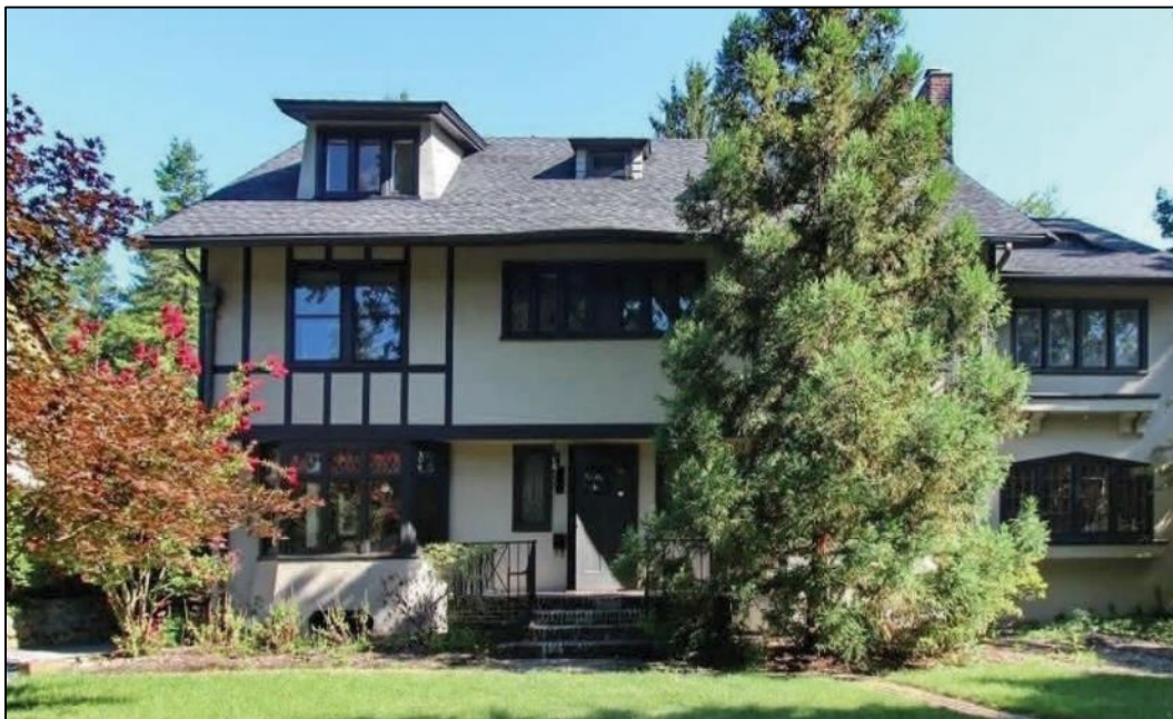
Figure 80 - Craftsman dwelling at 143 Gates Avenue, built in 1912. The dwelling has a stucco exterior with half-timbering.
