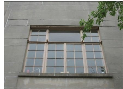
Figure 123 - Original steel casement windows at 20 Church Street.
