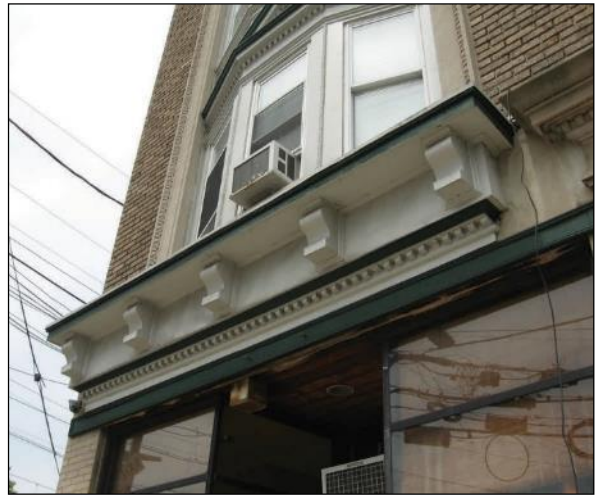
Figure 35 - Buildings in the Pine Street Historic District display notable detailing such as this storefront cornice at 43 Glenridge Avenue
