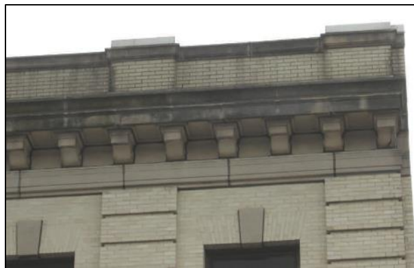
Figure 104 - Concrete cornice at 294 Bloomfield Avenue.
