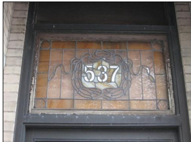
Figure 97 - The distinctive stained glass transom over the entrance of 537 Bloomfield Avenue is intact and not concealed.
