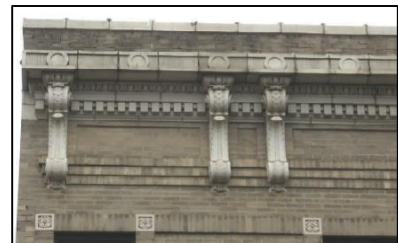
Figure 132 - A sheet metal cornice at 401 Bloomfield Avenue.
