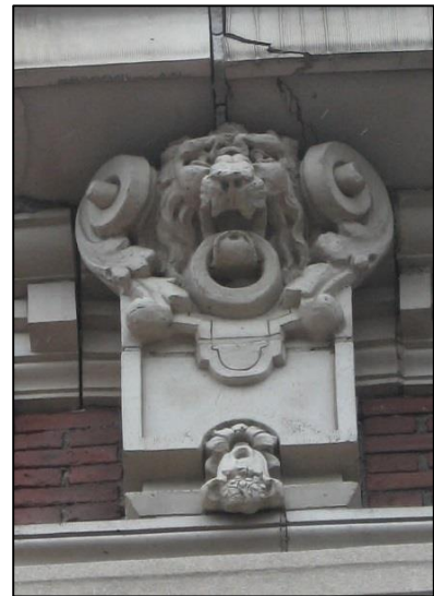
Figure 128 - Preserve and maintain original architectural details such as at 613 Bloomfield Avenue
