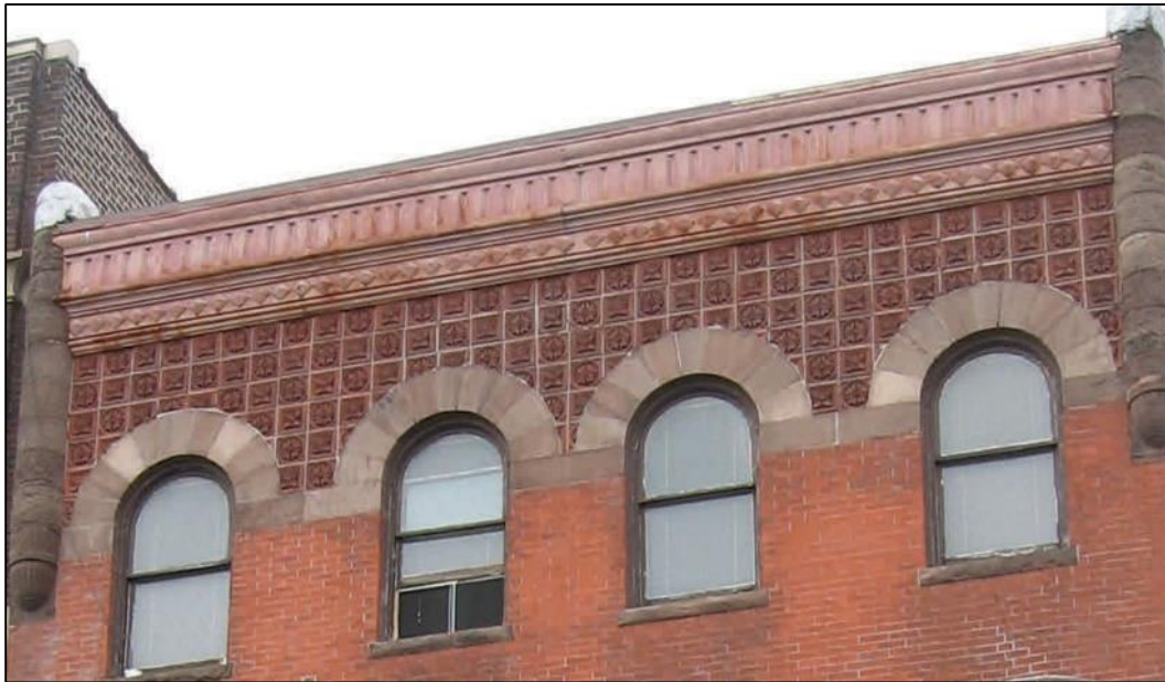
Figure 62 - Upper floor detail of the building at 425 Bloomfield Avenue.
