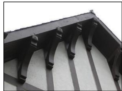
Figure 134 - Gable roofs are not as common as flat roofs in commercial streetscape and should be preserved, along with their decorative features such as brackets at 620 Valley Road.
