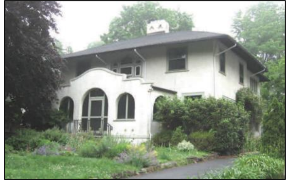
Figure 77 - The dwelling at 31 Fairfield Street is an example of the Mission style and has a stucco exterior and curvilinear parapet on the projecting front porch.
