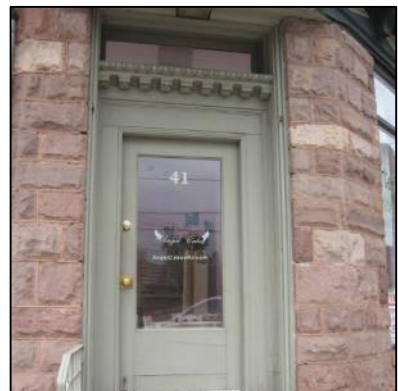
Figure 95 - Original door and transom at 41 Glenridge Avenue.
