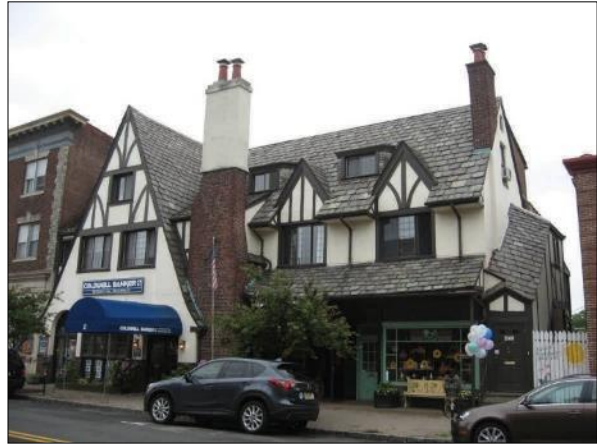
Figure 5 - Design guidelines help to ensure that historic buildings such as the commercial building at 242 Bellevue Avenue retains its historic character while it continues to be an asset to Montclair.
