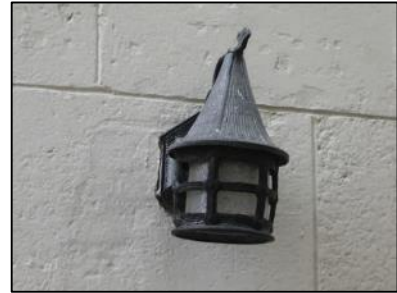
Figure 100 - Original light fixture at 42 Church Street.
