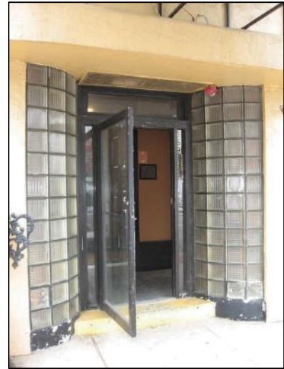
Figure 113 - Glass block entrance at 396 Bloomfield Avenue.
