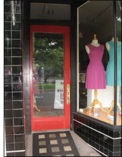
Figure 92 - Original, single-light door at 43 Watchung Plaza.
