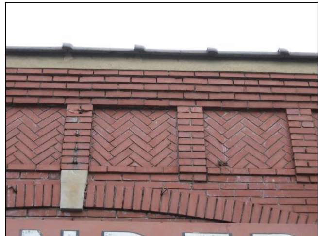
Figure 117 - Unpainted masonry should be left unpainted. Adding paint to this building would obscure its original texture, colors and details (627 Valley Road).
