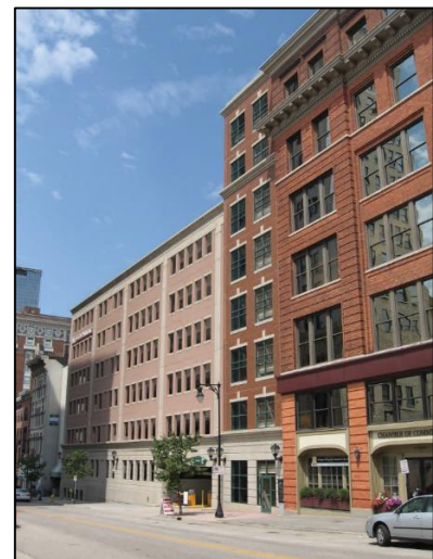
Figure 159 - The modern parking garage at the left in the photo was designed to complement the adjacent historic structures and be consistent with door and window openings.
