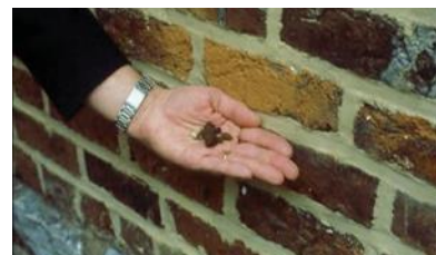
Figure 109 - Hard impermeable modern mortars (shown above) may force moisture through the more permeable brick and force mechanical stresses to be relieved through the softer brick which may lead to cracking, spalling, and erosion (shown below)
