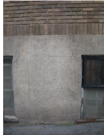
Figure 140 - Original concrete foundation at 6-9 Park Street.
