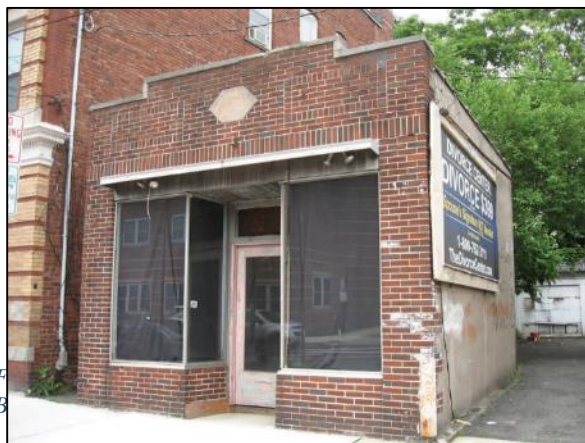
Figure 40 - The one-story building at 190A Bloomfield Avenue is an example of One-Part Commercial Block
