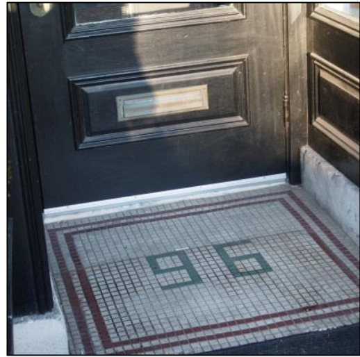
Figure 50 - Entryway tile at 96 Walnut Street
