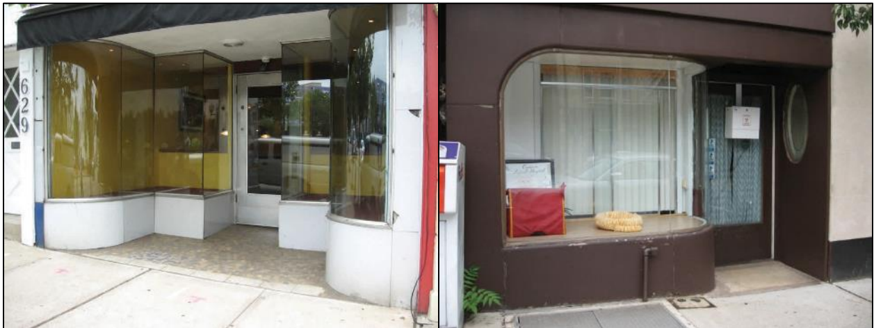
Figure 82 - The building storefront at 419 Bloomfield Avenue (right) features curved window frames and bulkheads and a circular window representative of the Art Moderne style. At left is a similar Art Moderne design, located at 629 Bloomfield Avenue
