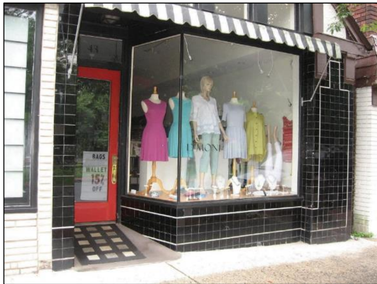
Figure 89 - This original storefront at 43 Watchung Plaza features many original elements, including its door and transom, display windows, and glazed tile bulkheads. An appropriate canvas awning has been added.
