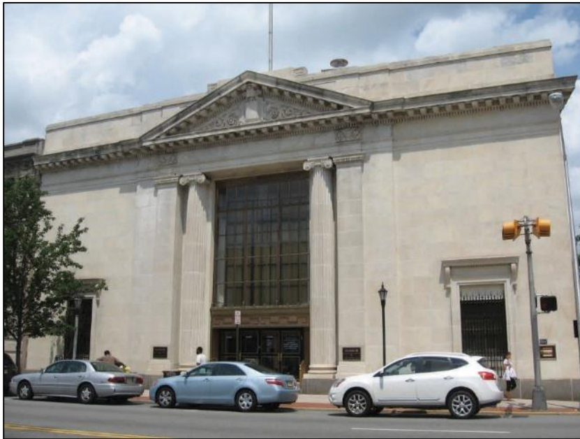
Figure 69 - The Chase Bank at 475 Bloomfield Avenue features a prominent portico at the entrance with Ionic columns.
