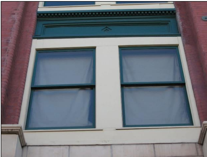
Figure 124 - These one-over-one sash windows are a good example of replacement windows. They match the historical design and configuration of the original windows.
