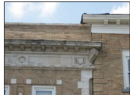
Figure 12 - Significant character includes decorative treatments on upper facades such as the cornices at 20 Lackawanna Plaza.
