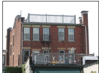
Figure 145 - Appropriate rear and roof decks at 621 Valley Road.
