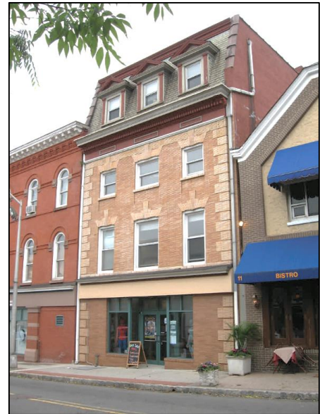
Figure 58 - This example of the Second Empire style illustrates the hallmark Mansard roof. The building's windows have decorative jack arches (9 S. Fullerton Avenue).
